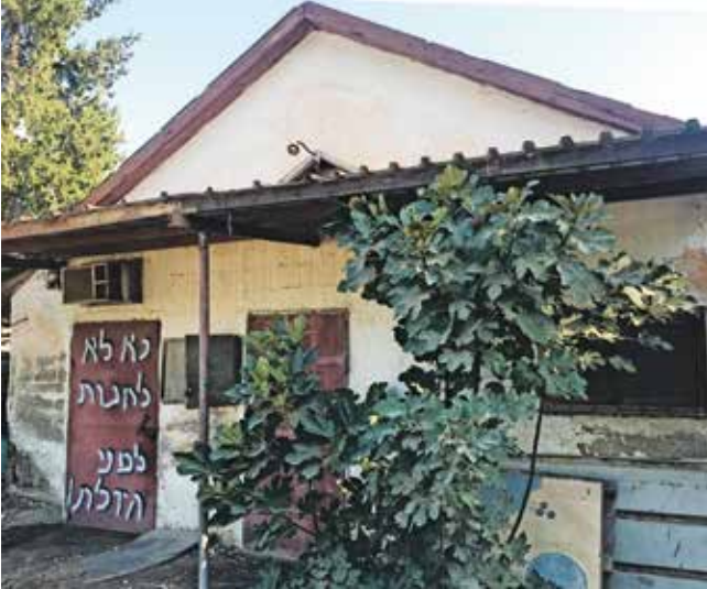
Illustration 2: Reusing an agricultural building, a barn that was repurposed into a youth club in Nahalal. Photo: Irit Amit-Cohen
